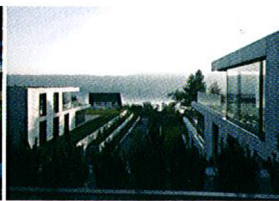
Residential Building Belsit Herrliberg CH
